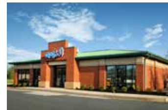
Riverside Branch 1327 Riverside Parkway Belcamp, MD
